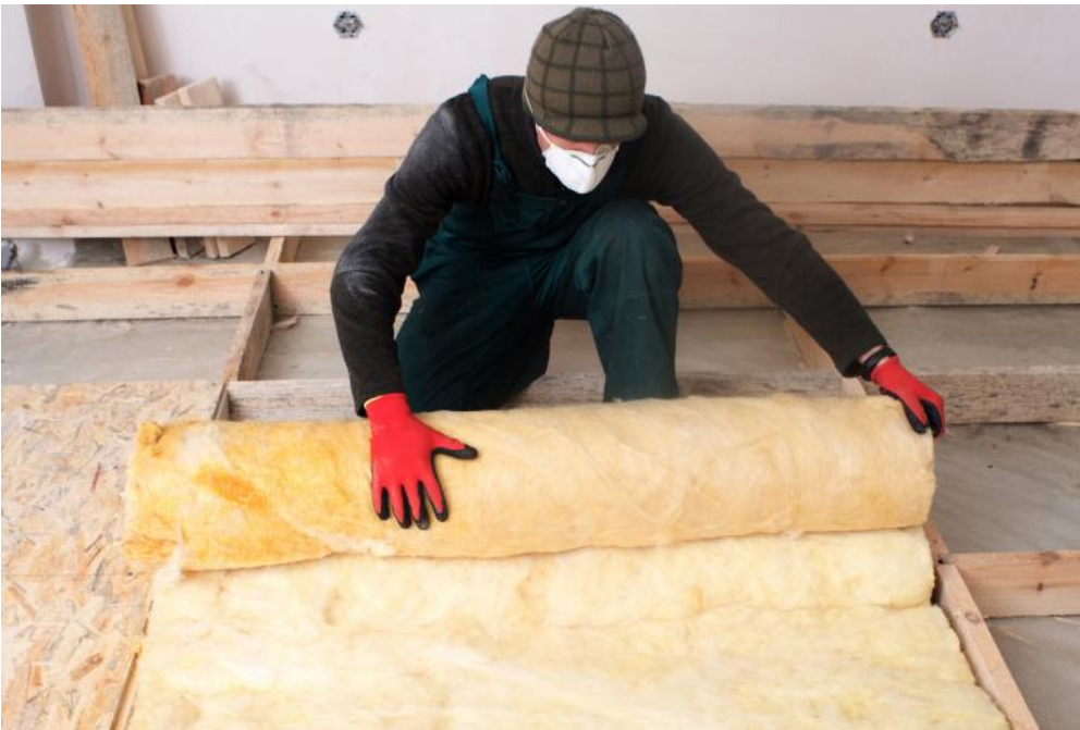
Home floor insulation. Photo: Shutterstock.com
