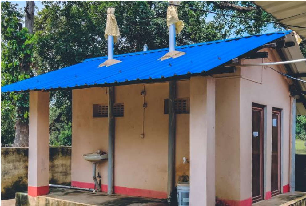
Community toilet in India.
