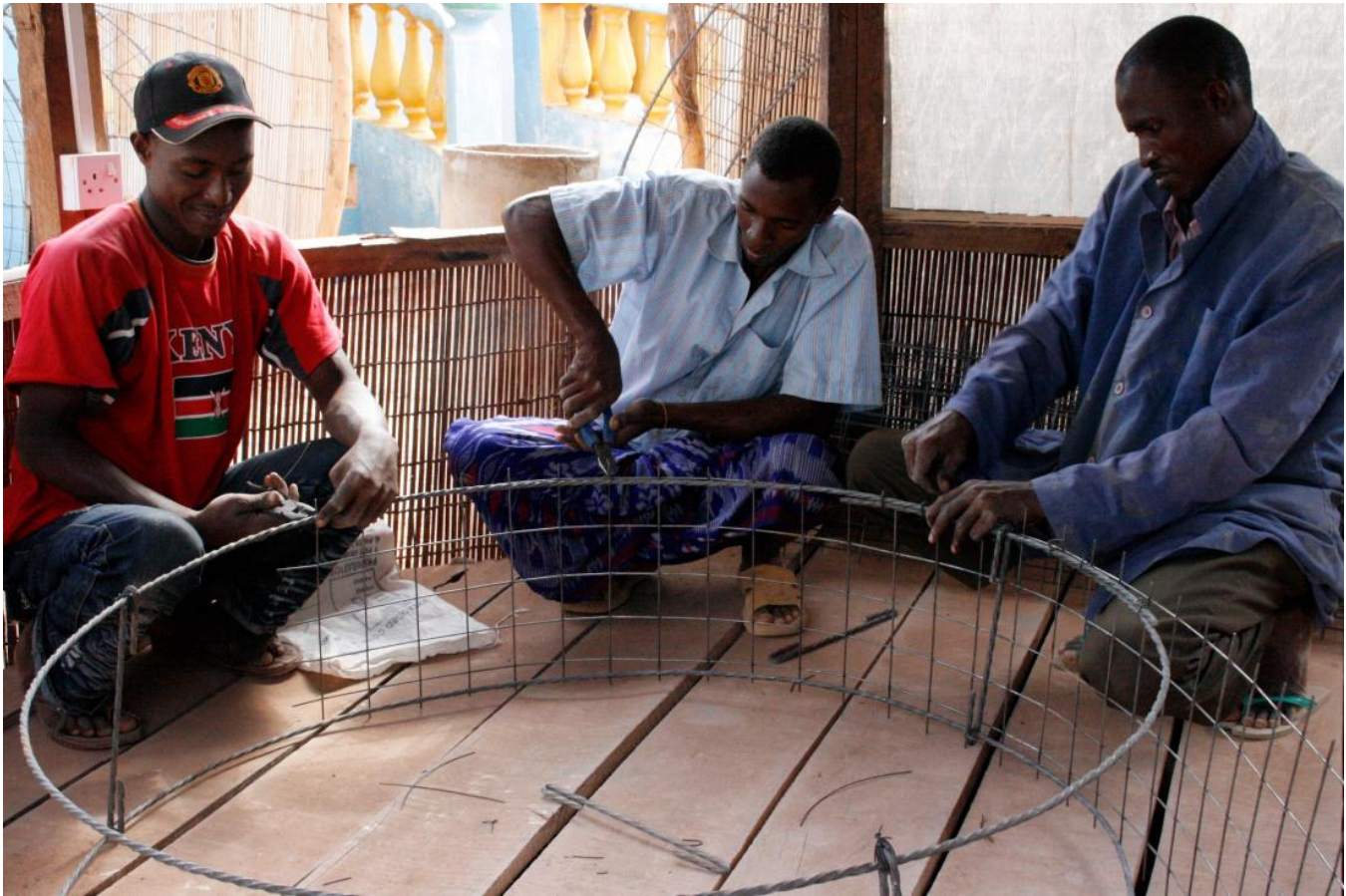
Three men assemble a metal well frame.
