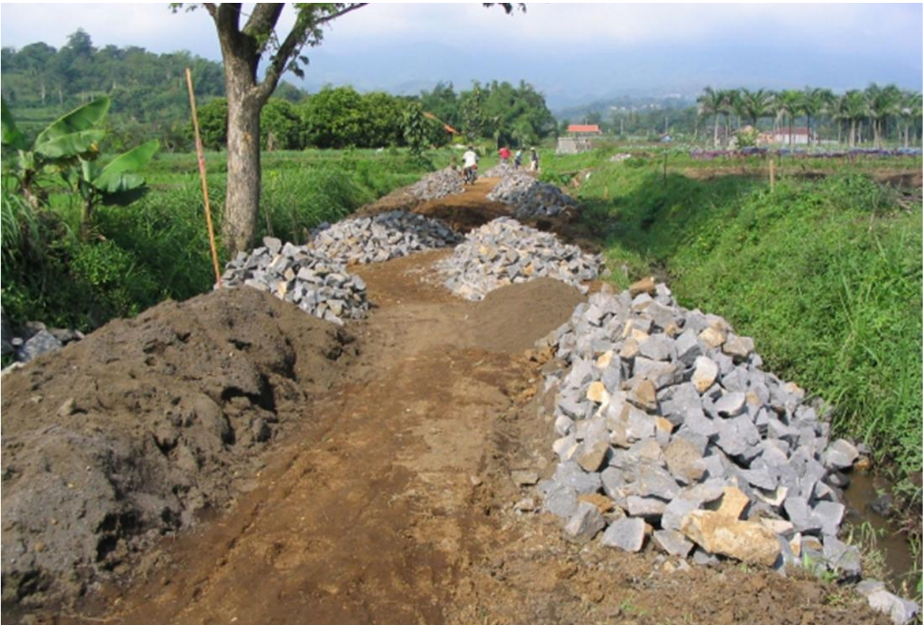
Road under construction in Indonesia.
