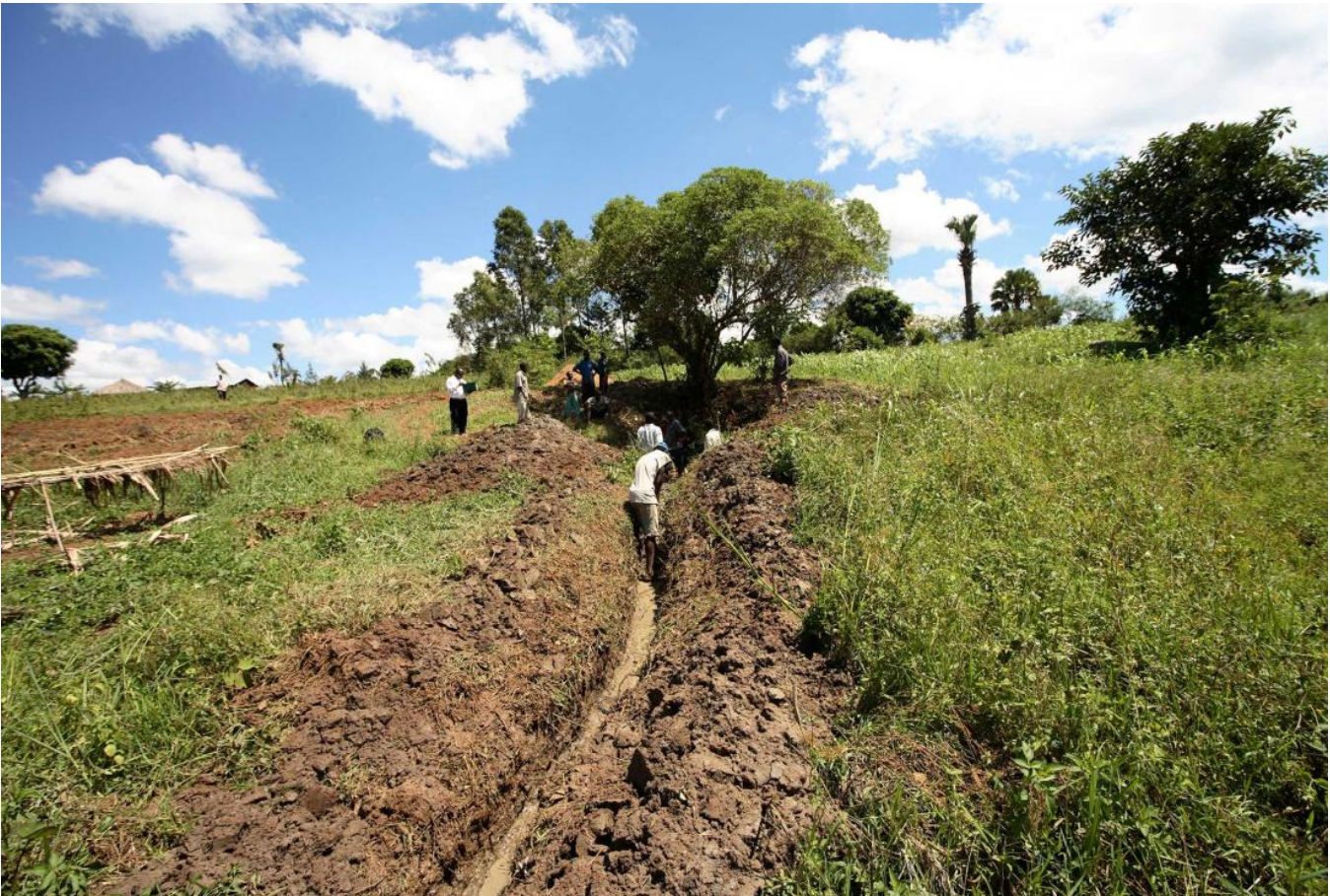
Introducing irrigation to central Kenya
