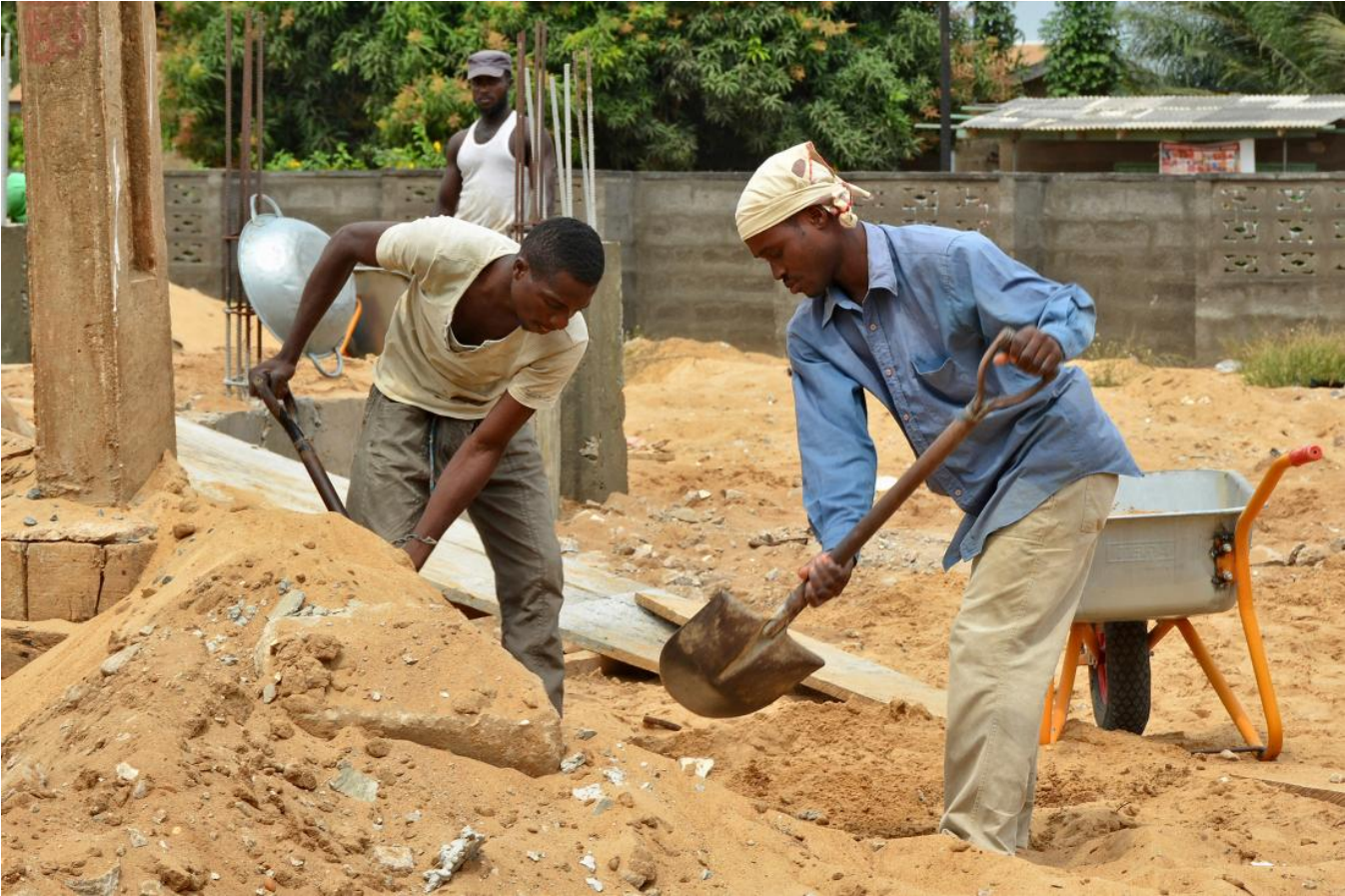
Workers complete a construction project.
