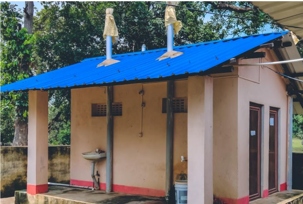
Community toilet in India.
