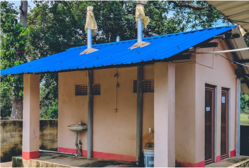
Community toilet in India.
