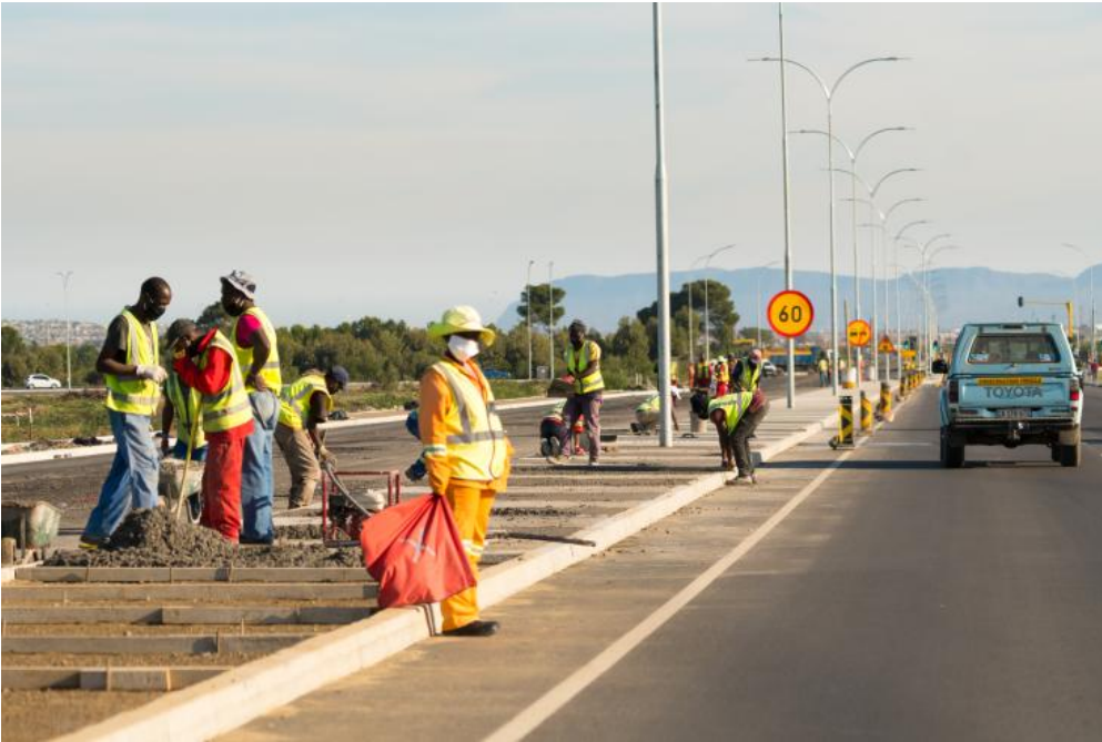
Construction workers build a road in Cape Town, South Africa
