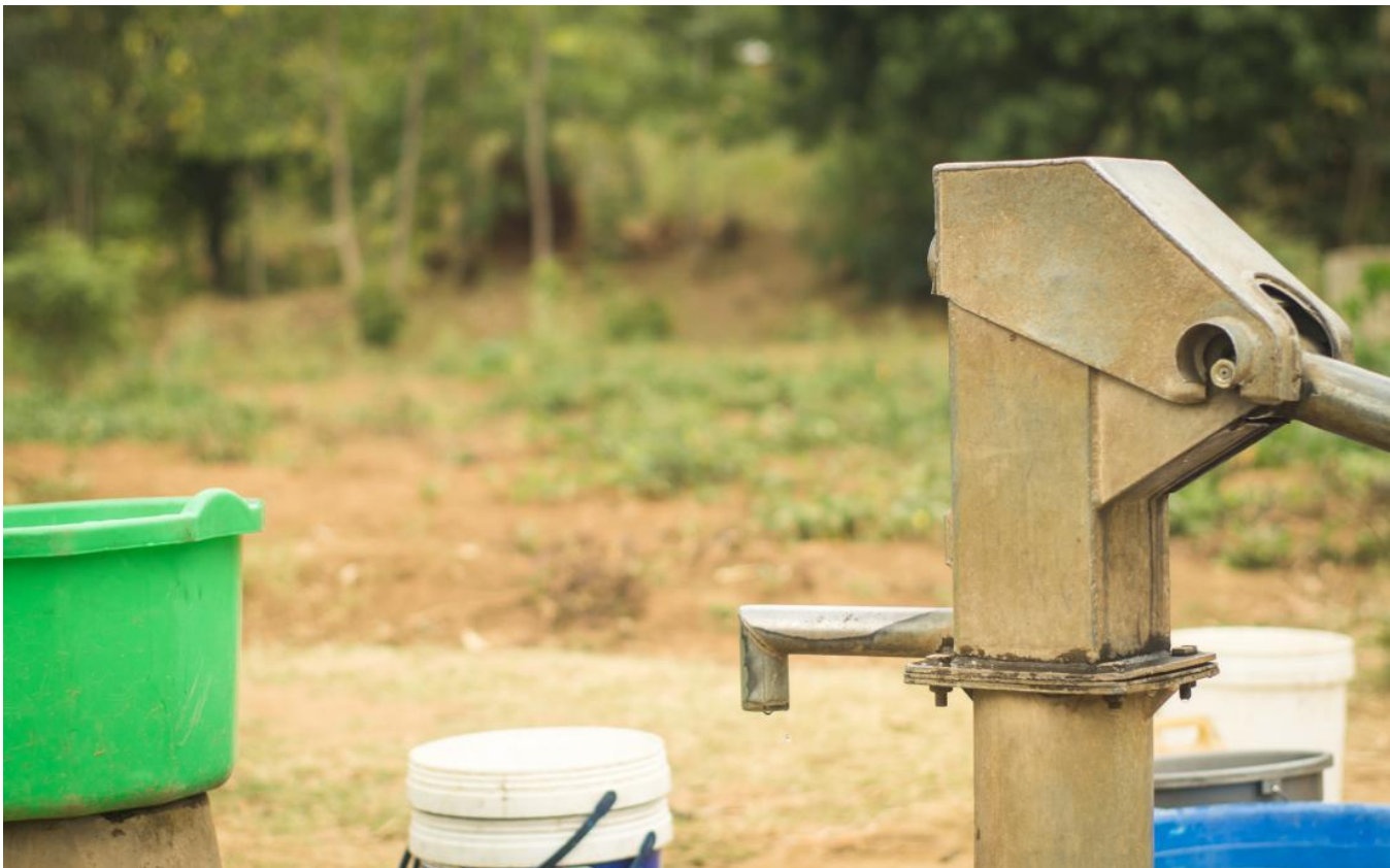
A water point in Malawi.
