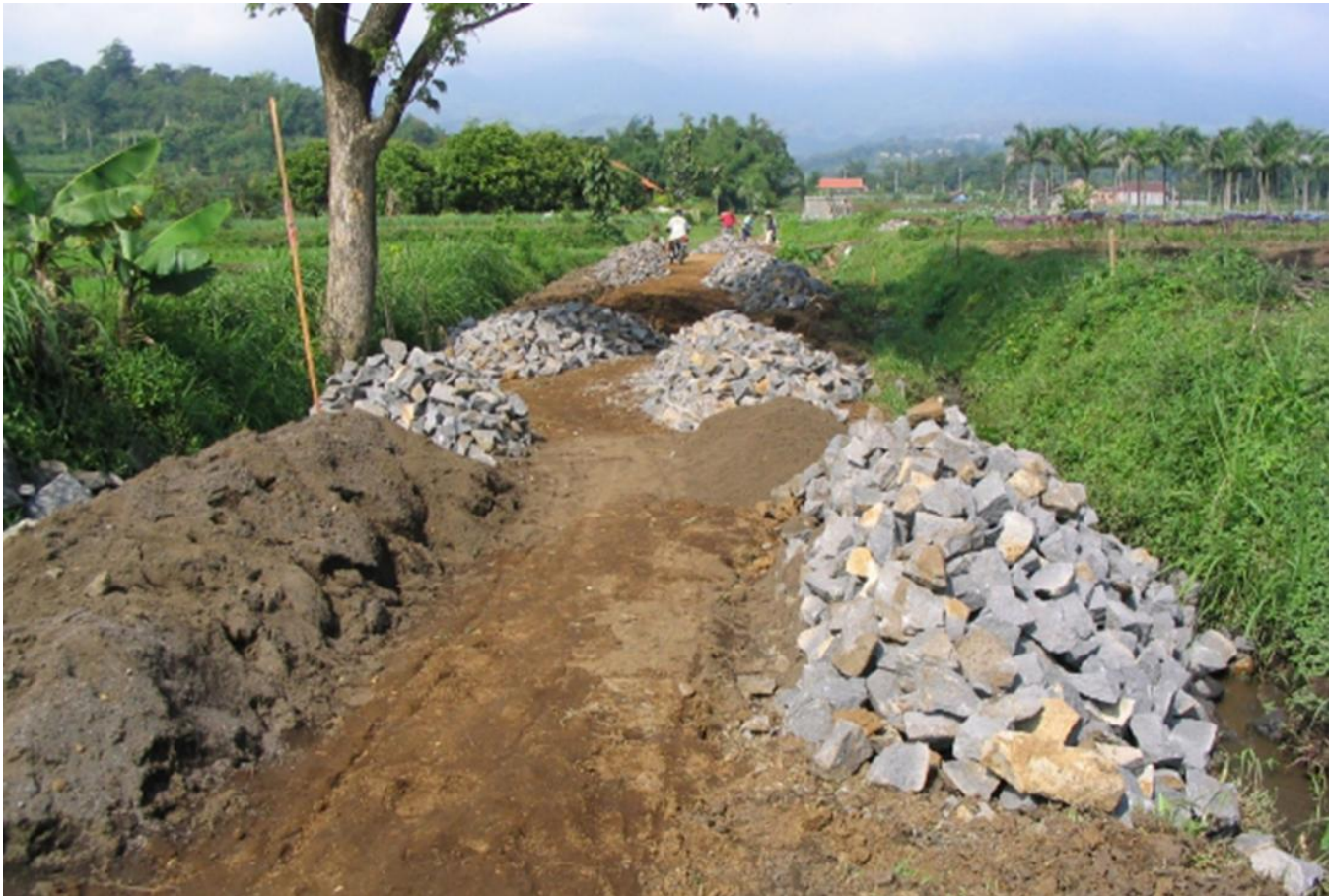
Road under construction in Indonesia.
