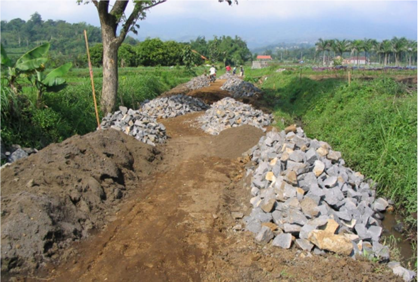
Road under construction in Indonesia.
