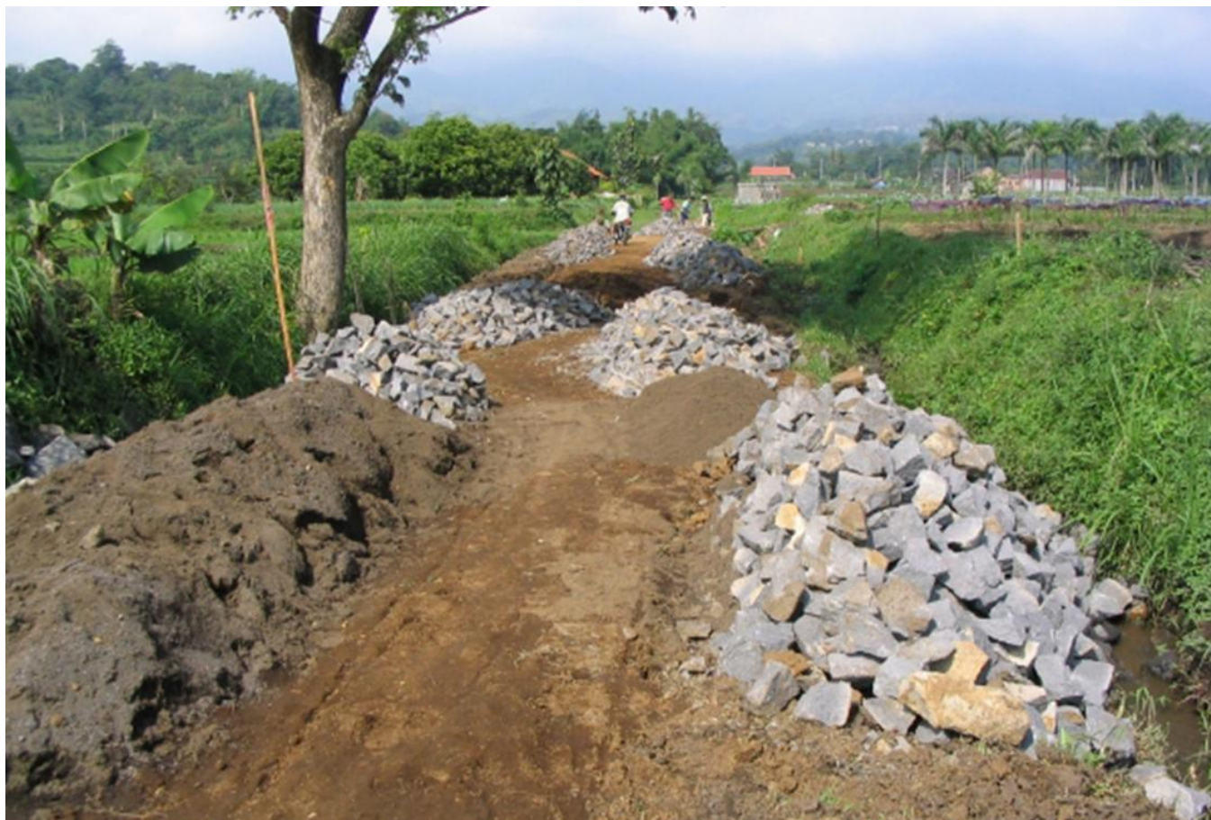
Road under construction in Indonesia.
