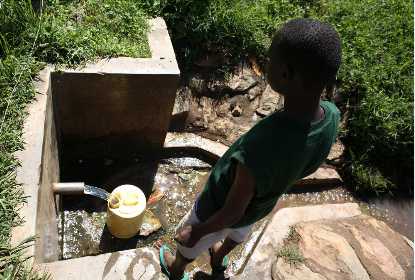
Boy watching water pour out of a concrete-encased spring.
