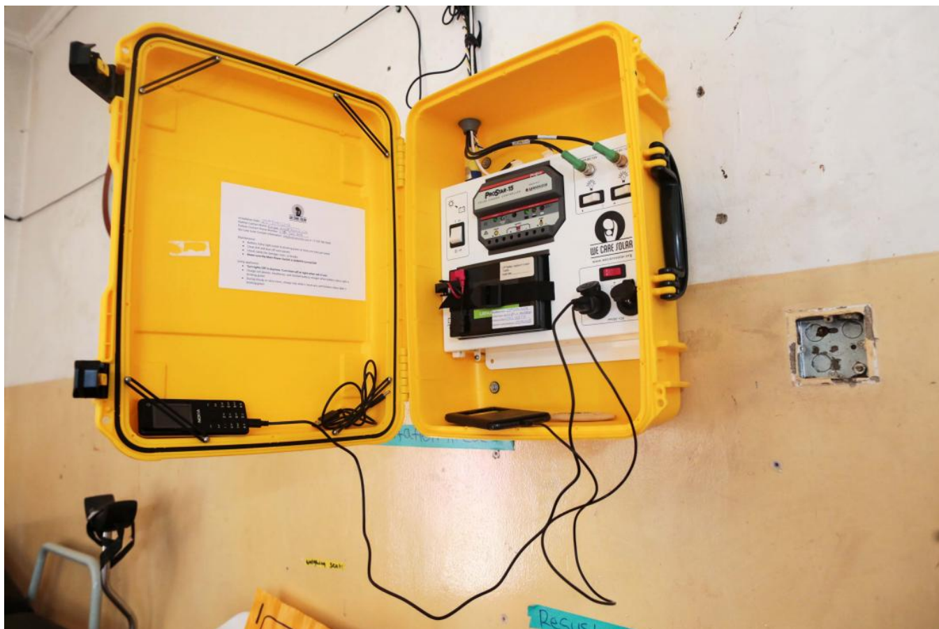
We Care Solar Suitcase® installed in a maternity care facility.
