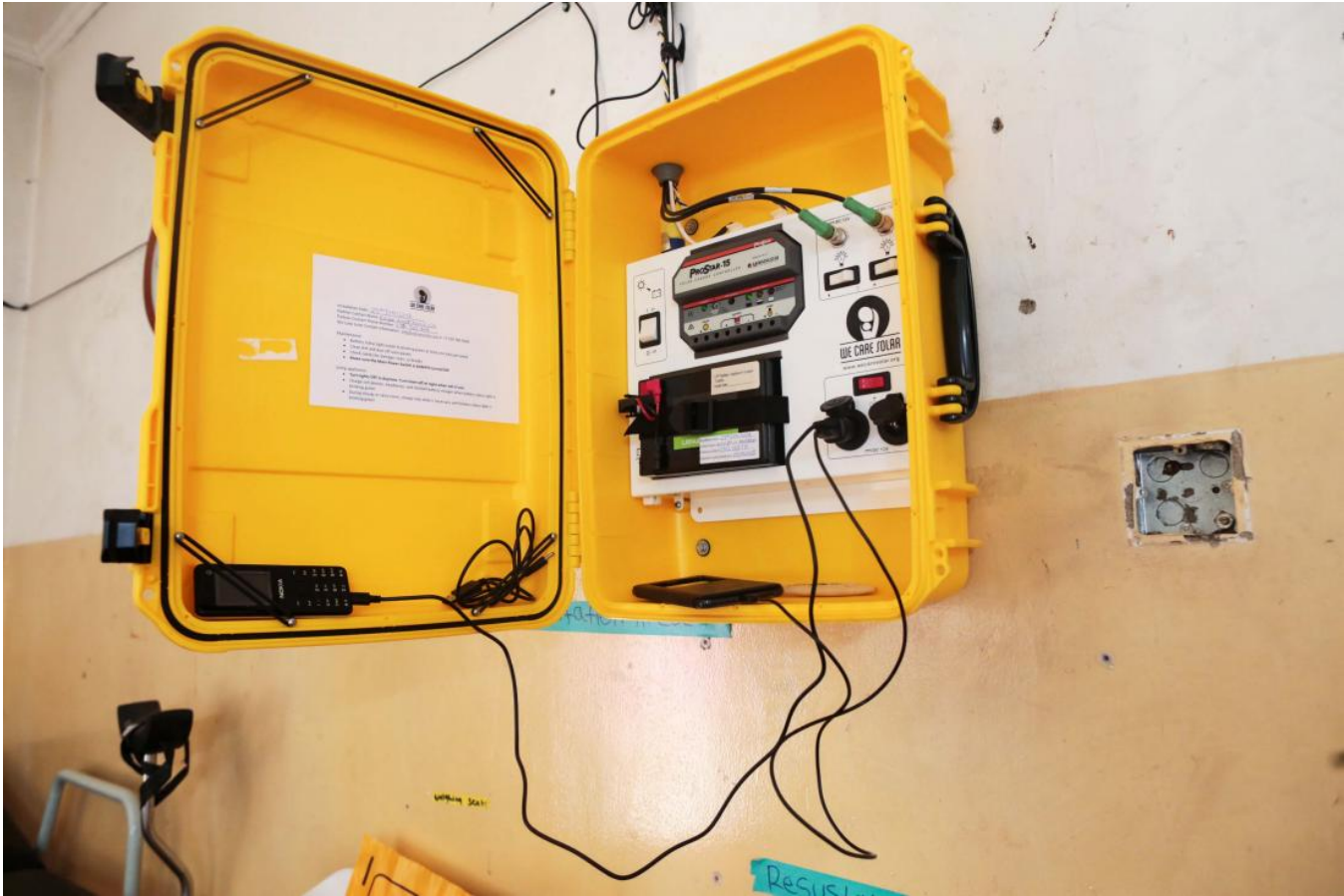
We Care Solar Suitcase® installed in a maternity care facility in Uganda.
