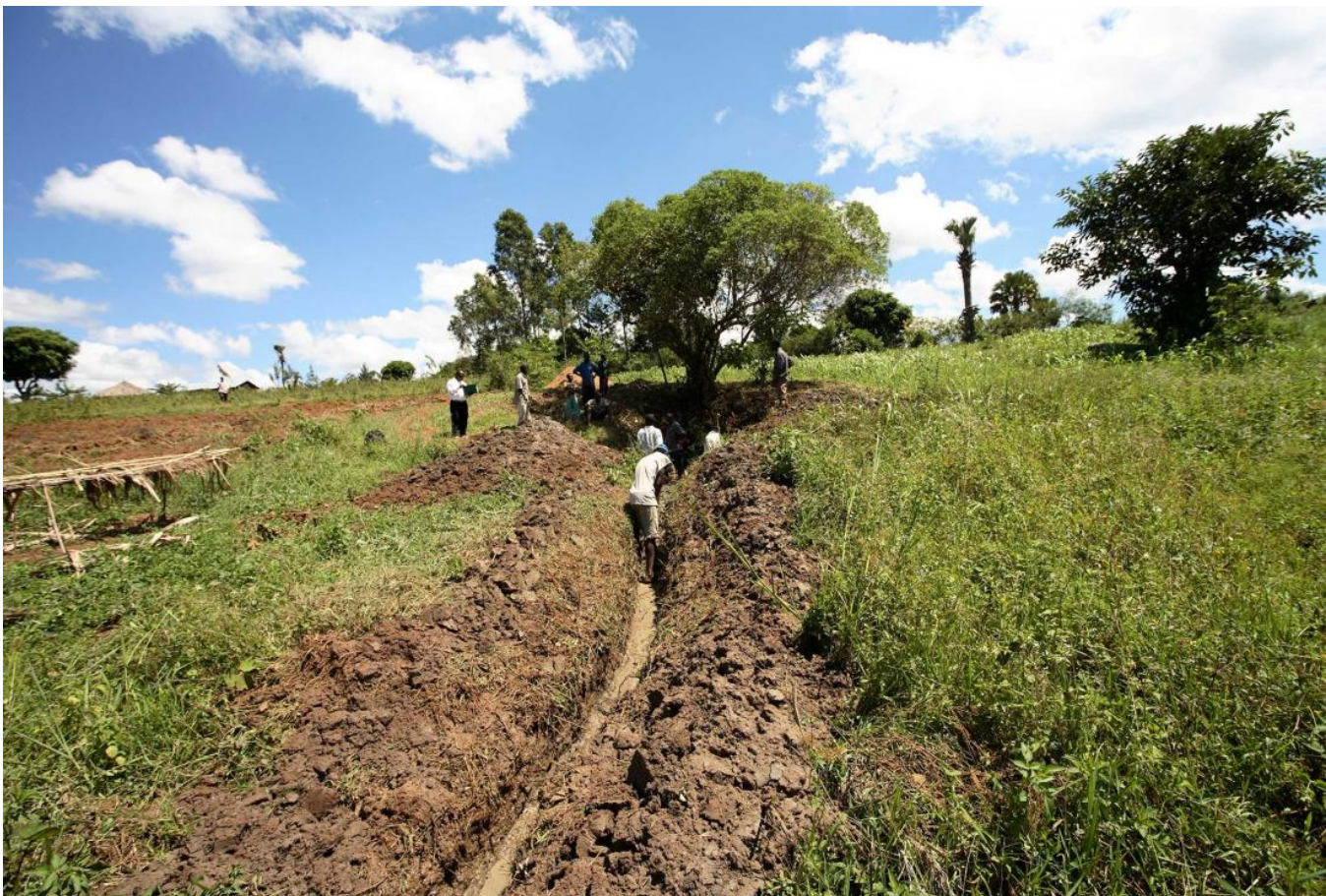
Introducing irrigation to central Kenya
