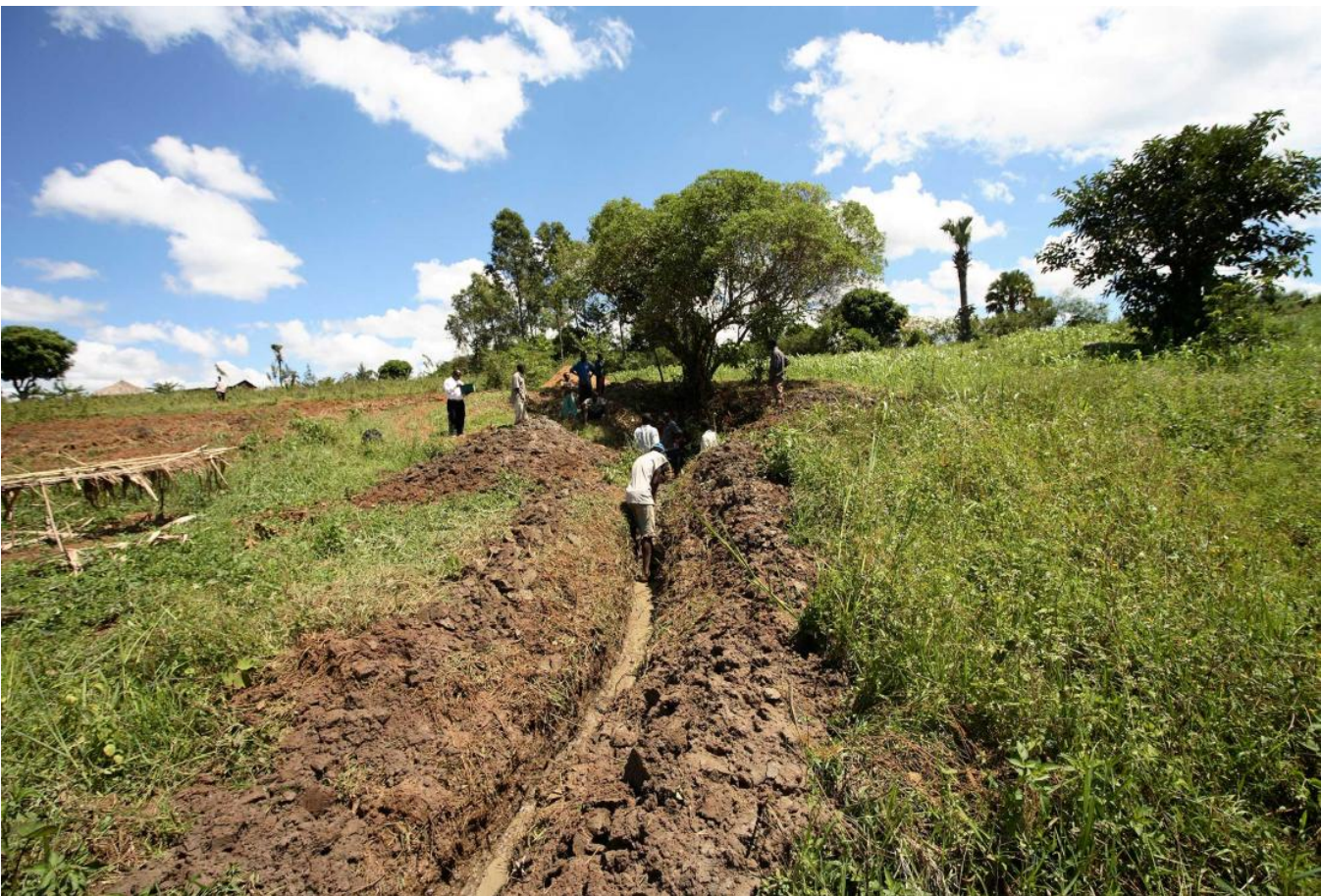
Introducing irrigation to central Kenya
