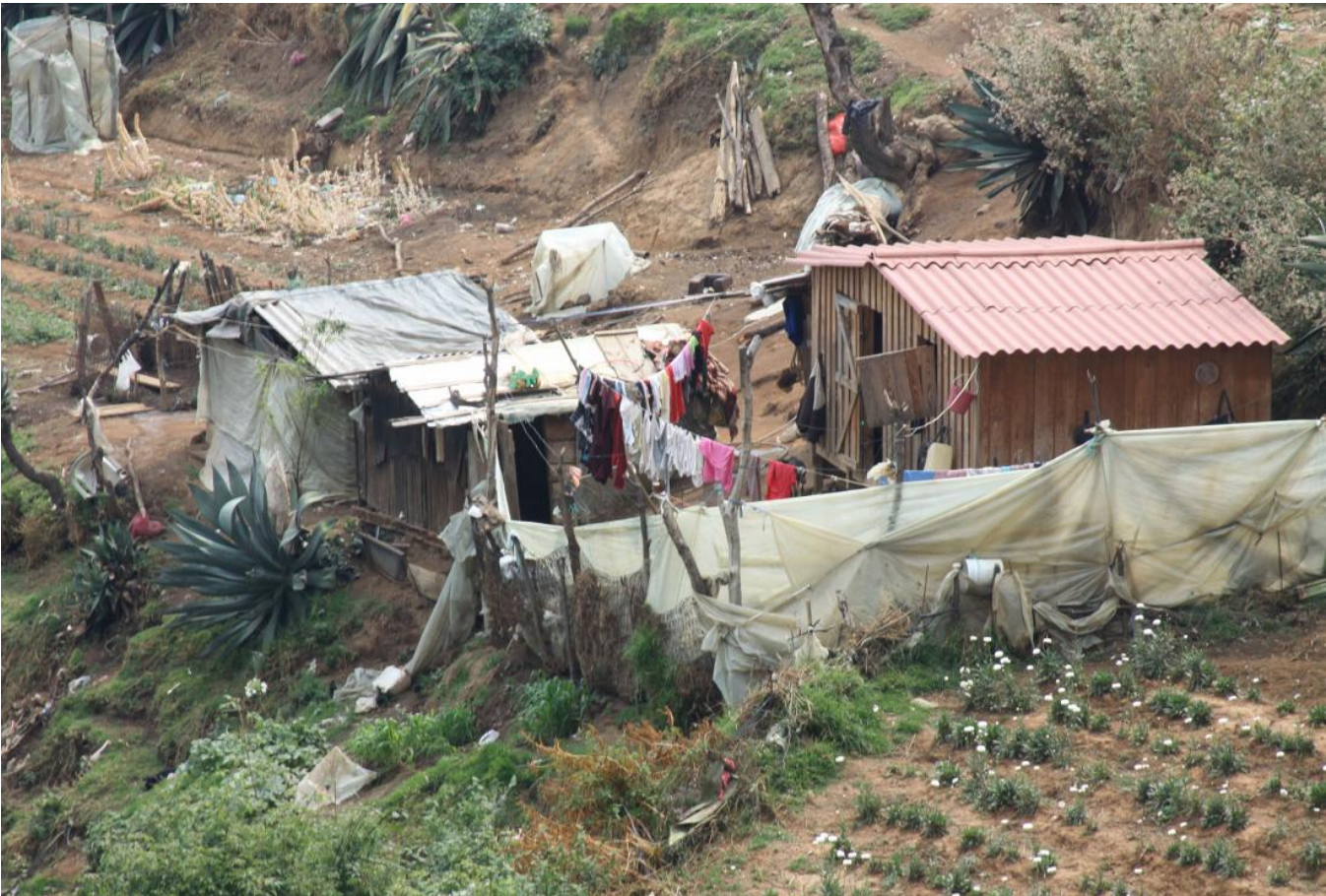
Slum housing in Mexico
