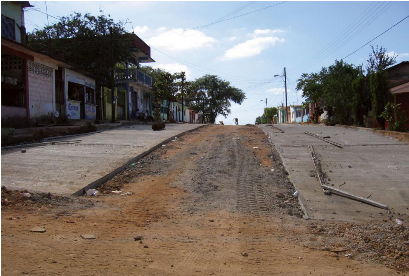
Road being paved in Acayucan, Mexico
