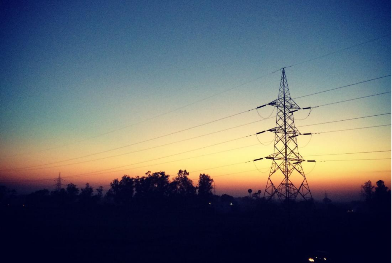
A power tower supports electrical lines in Bihar, India. Photo: Prianthi Roy | J-PAL
