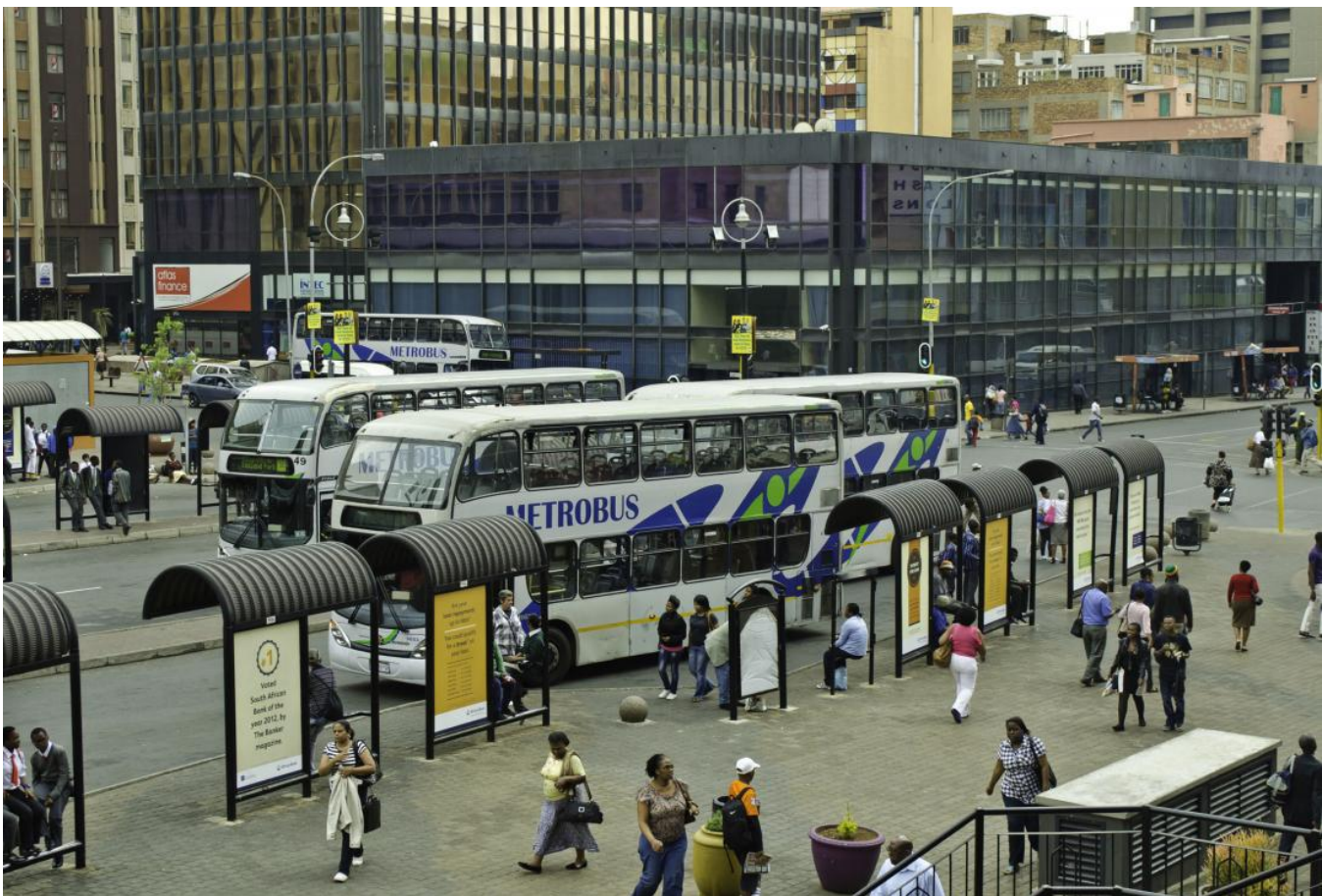
Bus station in South Africa
