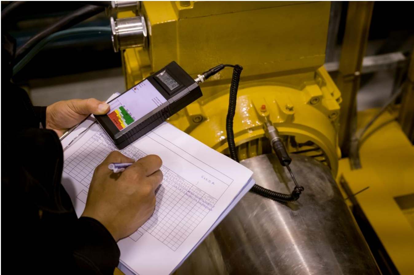
Technician inspecting a power plant, India.
