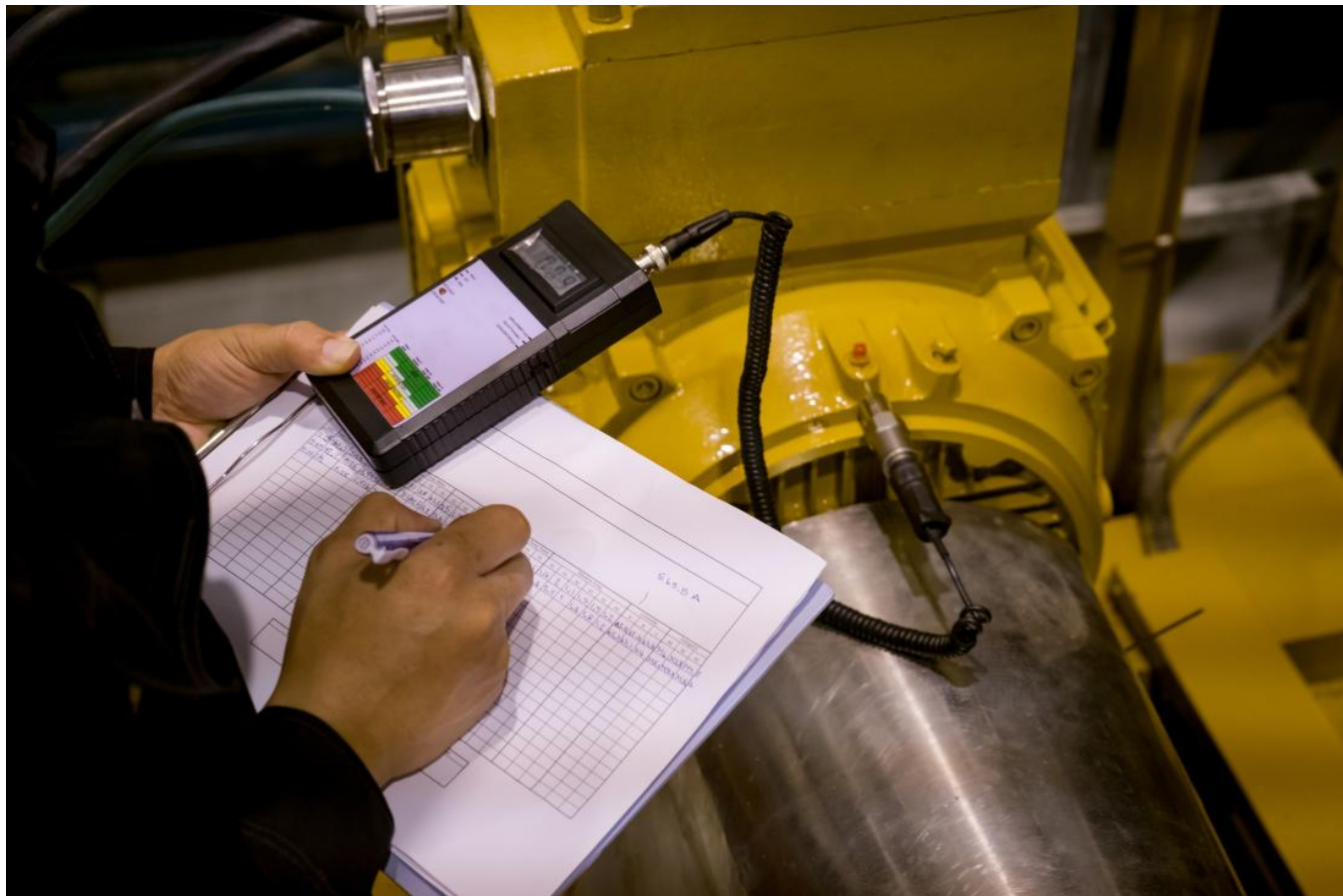
Technician inspecting a power plant, India.
