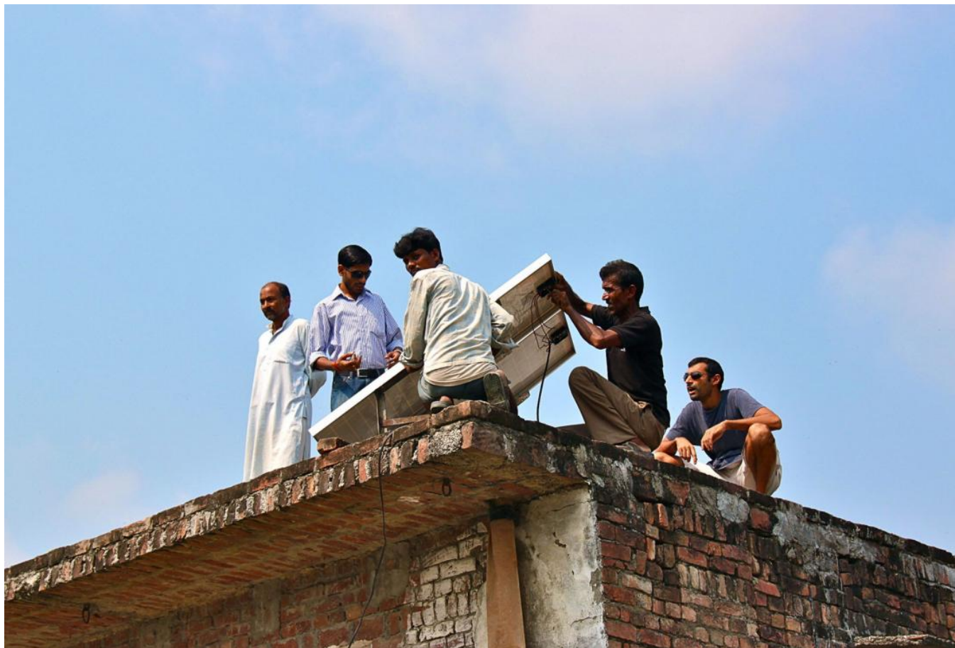
Installing a solar microgrid in India. Photo: Anna da Costa | CC BY-NC-ND 2.0
