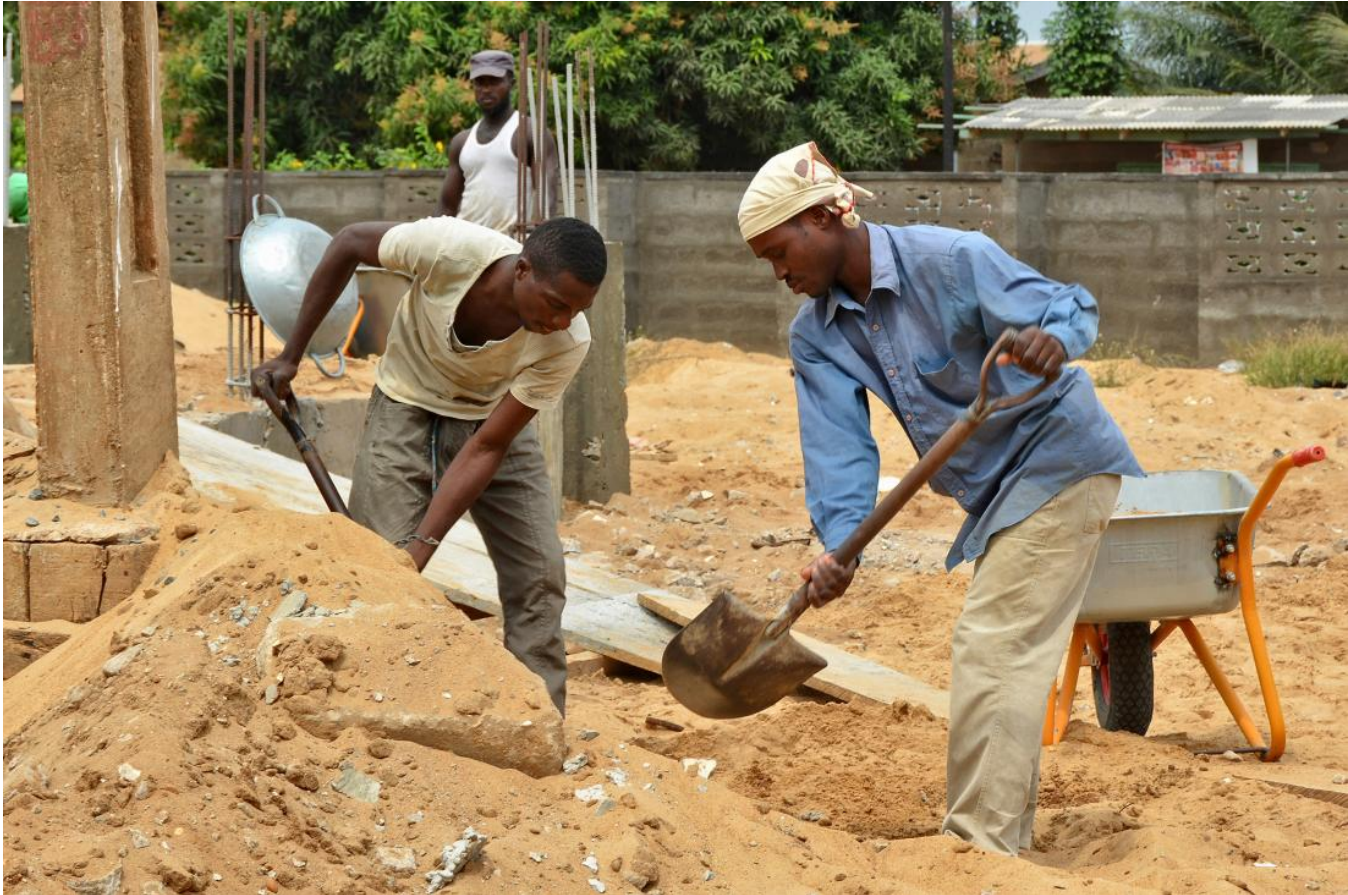
Workers complete a construction project.
