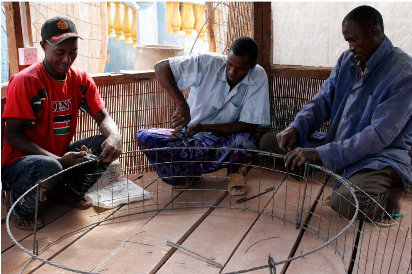
Three men assemble a metal well frame.
