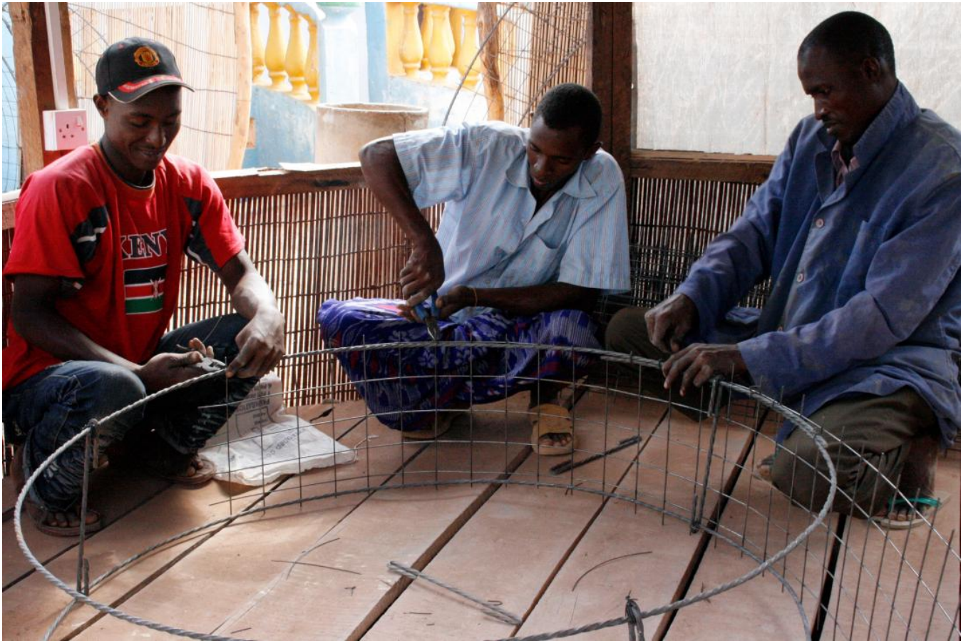
Three men assemble a metal well frame.
