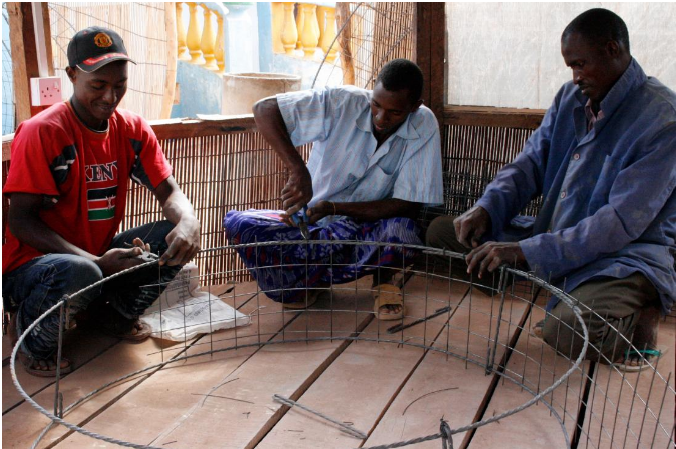
Three men assemble a metal well frame.
