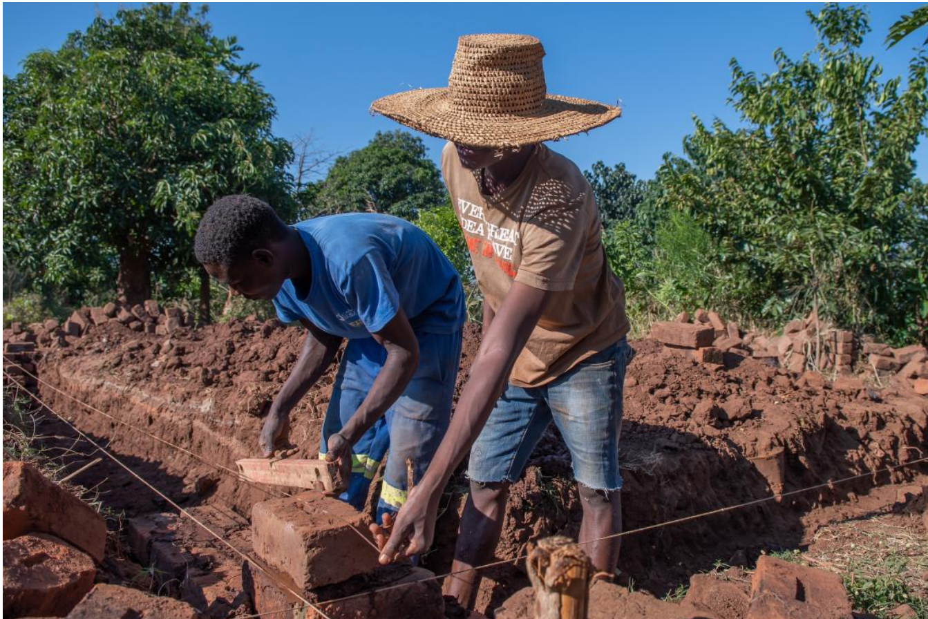
Young farmers construct an exterior wall of a home in Malawi.
