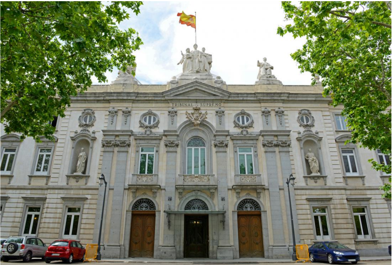
Supreme Court of Spain building in Madrid. Photo: Shutterstock.com
