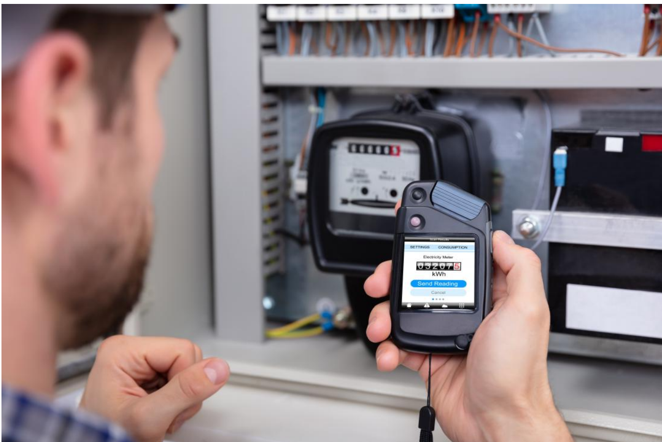
A technician reads a meter.
