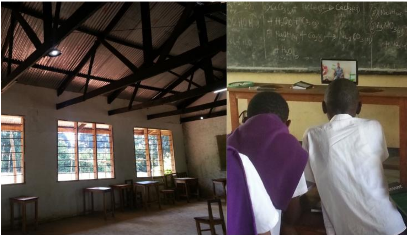
On the left, lights are installed in a classroom in Tanzania; on the right, students look at a screen at the front of the classroom delivering educational instruction.
