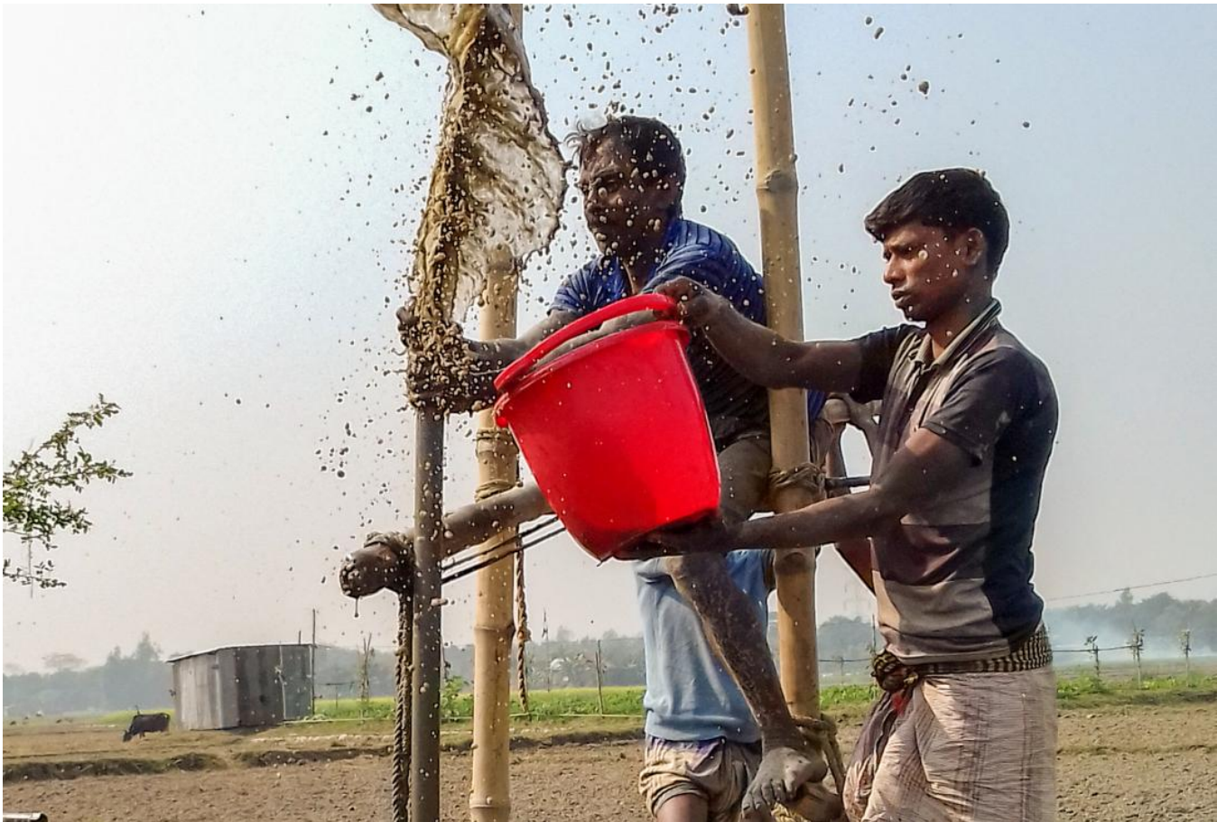
Drillers installing a private shallow well in Araihasar, Bangladesh. Photo: Alexander van Geen | J-PAL
