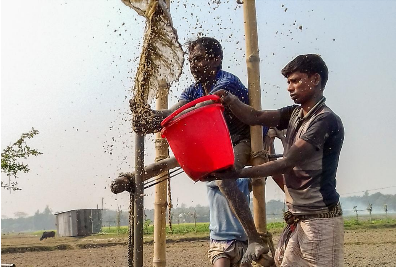
Drillers install a private shallow well in Araihasar, Bangladesh.
