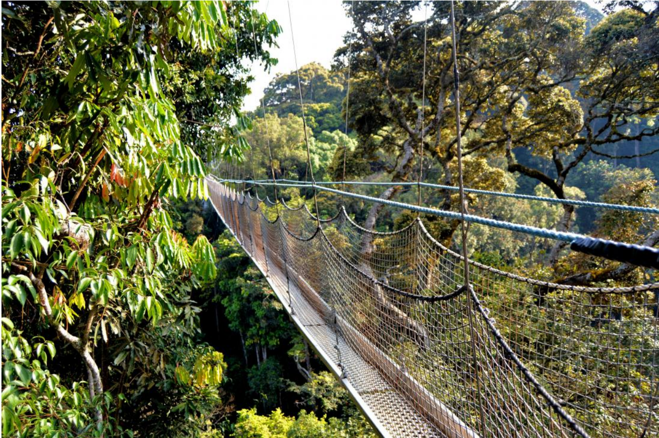
Footbridge suspended over a jungle in Rwanda.
