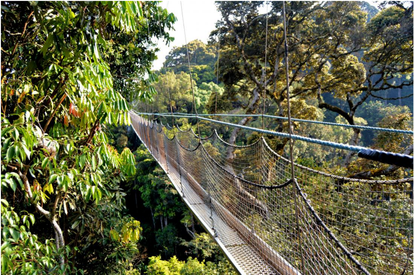
Footbridge suspended over a jungle in Rwanda.
