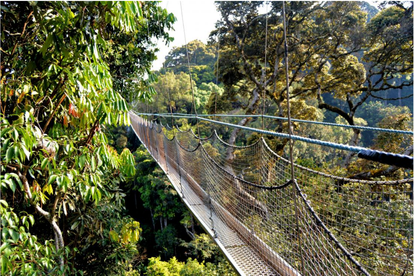
Footbridge suspended over a jungle in Rwanda.
