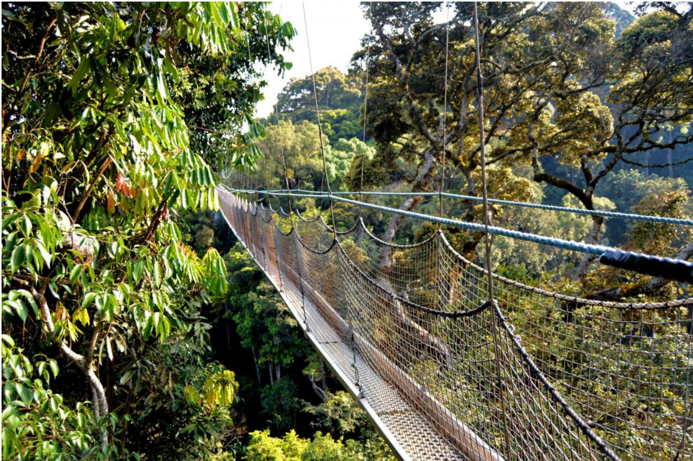
Footbridge suspended over a jungle in Rwanda.
