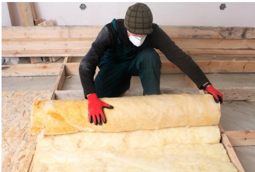
Home floor insulation. Photo: Shutterstock.com
