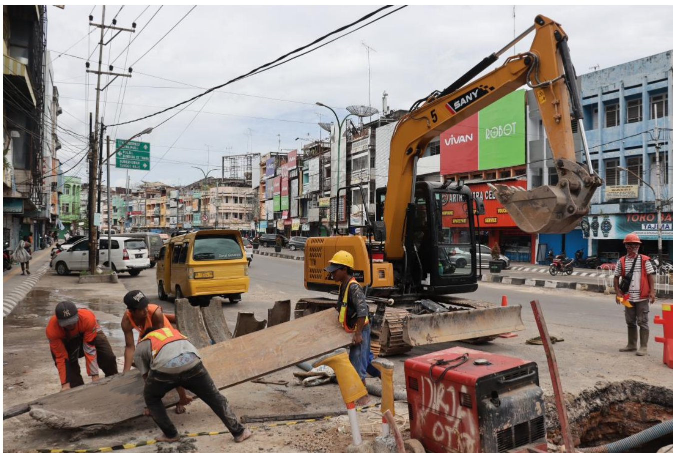
Seasonal Migrant workers in Indonesia working in construction in urban environment.
