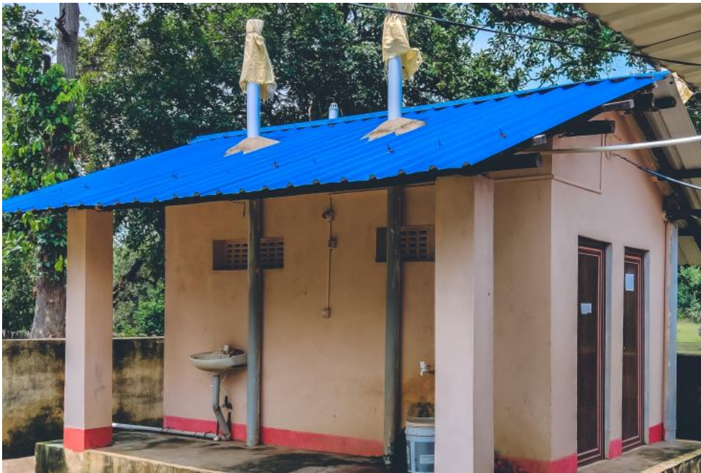
Community toilet in India.
