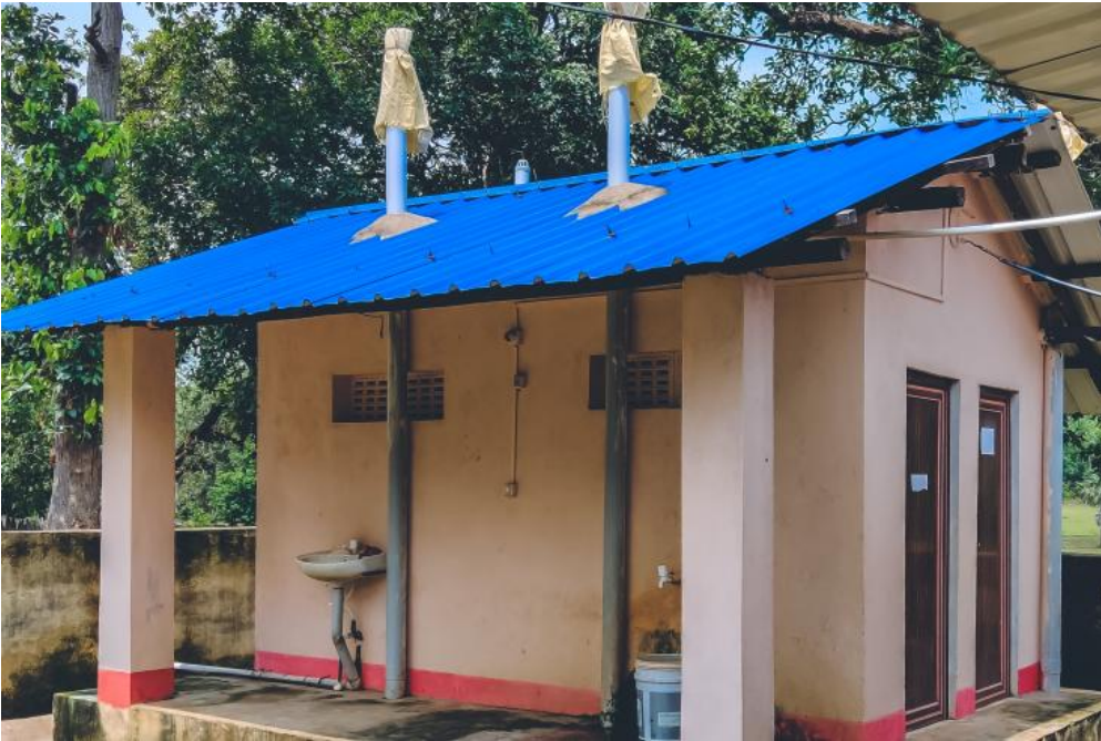
Community toilet in India.
