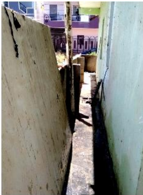
Passage after the intervention
