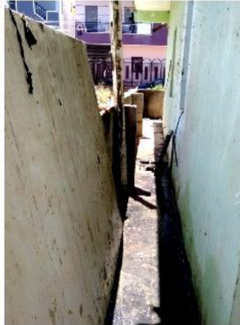
Passage after the intervention
