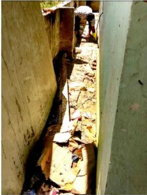
Passage before the intervention
