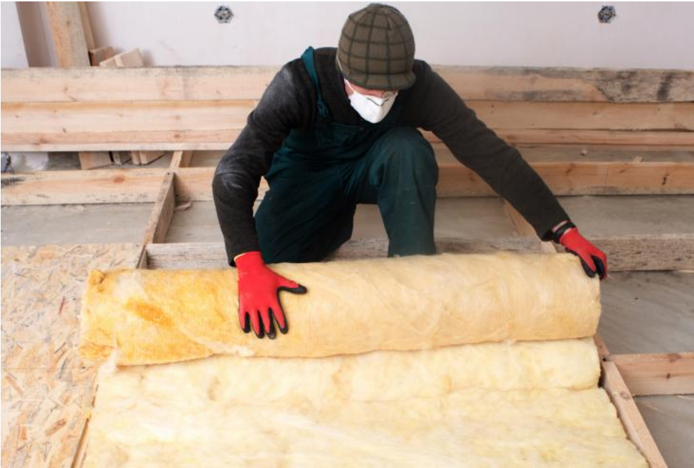
Home floor insulation. Photo: Shutterstock.com
