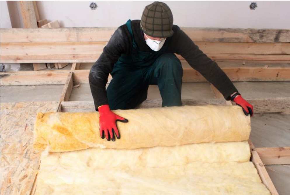
Home floor insulation. Photo: Shutterstock.com
