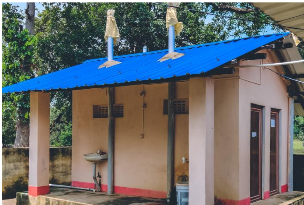
Community toilet in India.
