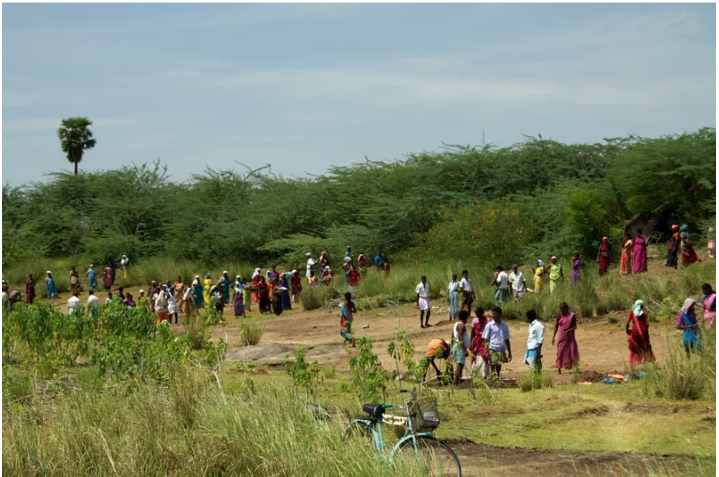
National Rural Employment Guarantee participants working on digging out a silted-up water tank. | McKay Savage
